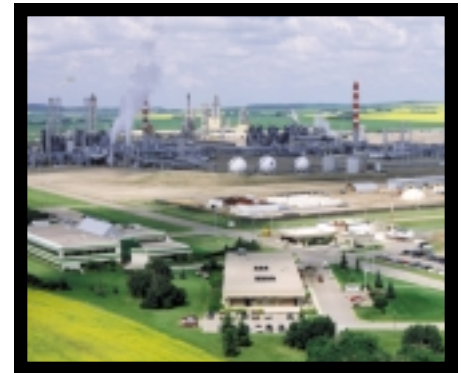
NOVA Chemicals Joffre, Alberta, Ethylene and Polyethylene production facility.
